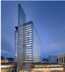
Manitoba Hydro Place
