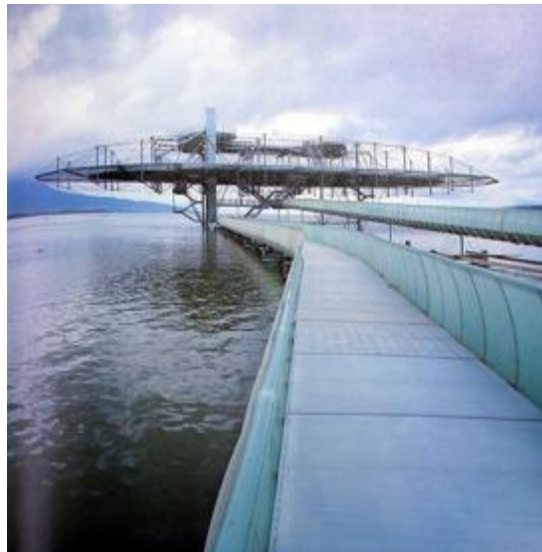
Figure 3: The Blur Building Before Fog Production. 7
